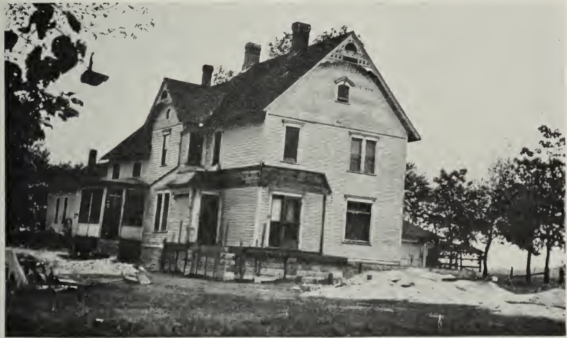
FIG. 41.—House near Coal City lowered 9 inches at one corner, caused by mining a 3-foot coal at a depth of 125 feet.
